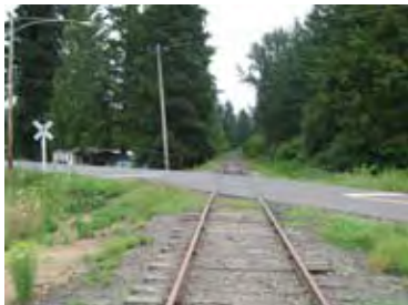
NE 259th Street crossing looking south.
