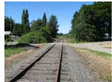
Driveway crossing north of NE Laurin Road near MP-8.5. The recommended alignment is left of track.
