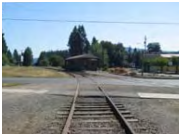
Yacolt Road crossing of the wye.
