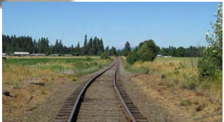
View near MP-8.7. Narrow 60-foot ROW and potential rail operations conflicts in area proposed for rezoning to Railroad Industrial will require coordination of trail alignment with development code and site design to maintain trail continuity.
