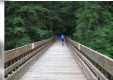
The trail bridge across East Fork Lewis River.
