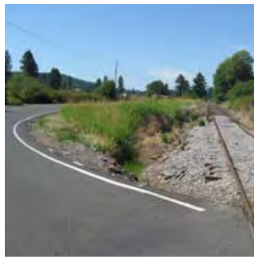
On grade crossing of NE Railroad Avenue south of Yacolt near MP-25.4.
