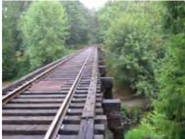
Trestle across Salmon Creek at MP-12.4.
