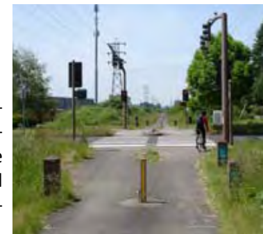
Properly located bollards approaching a Type II roadway crossing. Note the tall equestrian push button at right. Springwater Trail, Portland, OR.
