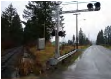
Limited sight distance and the diagonal crossing at NE 182nd Avenue.
