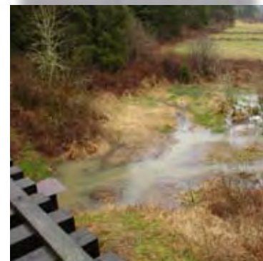
Trestle at MP-18.1 across a creek and wetlands.
