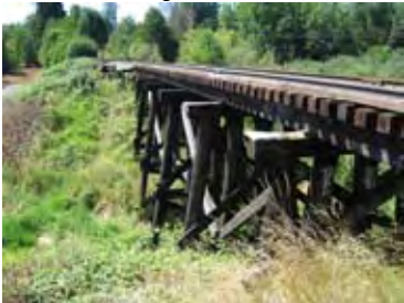
Curtin Creek Bridge at MP-6.5.
