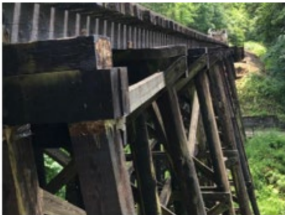
Bridge 12 at Salmon Creek has rotting and shifting timbers.
