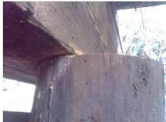
Bridge 12 at Salmon Creek has rotting and shifting timbers.
